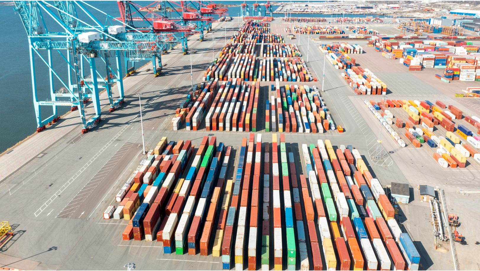
The Port of Gothenburg container terminal where the quay will be reinforced and the associated fairway deepened. This is to accommodate larger and heavier loaded vessels than what is possible today. Image: The Gothenburg Port Authority.
